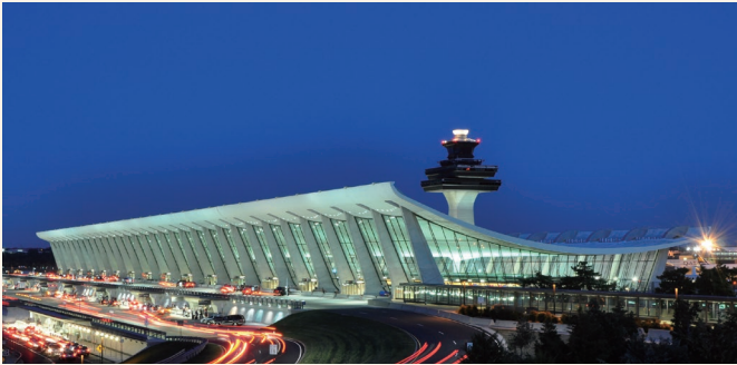
Fig.13: Washington Dulles International Airport [36] [37]
