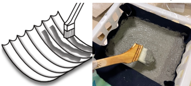
Fig4. Apply a thin layer of paint to the surface of the fabric form with a brush.
