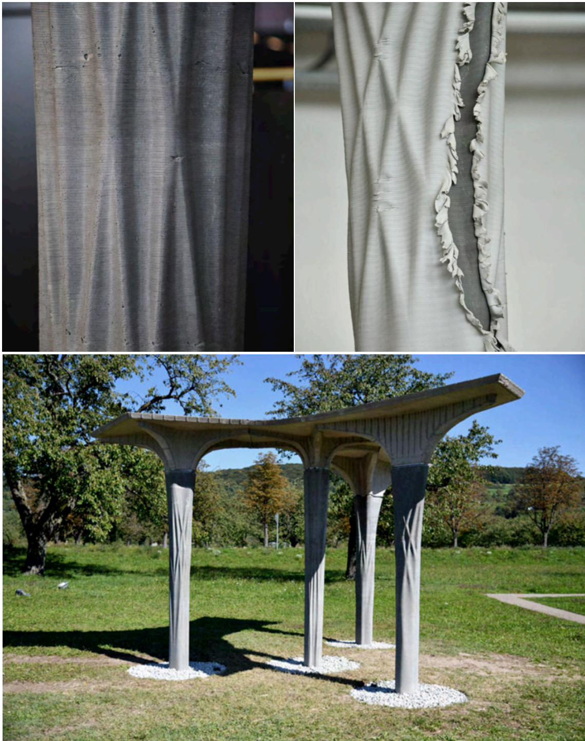
図 20: “eggshell pavilion”. ETH zurich explores digital design + robotic 3D printing in concrete .2022 ( https://www.designboom.com/architecture/eth-zurich-gramazio-kohler-digital-design-robotic-3d-printing-eggshell-pavilion-10-05-2022/ より引用)
